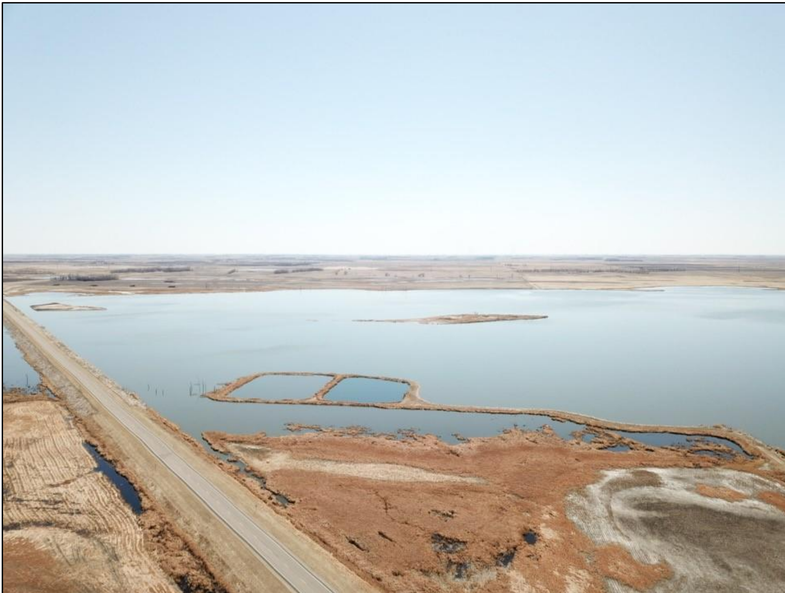
Figure 8.4.1 City of McHenry Sanitary Sewer Lagoons
