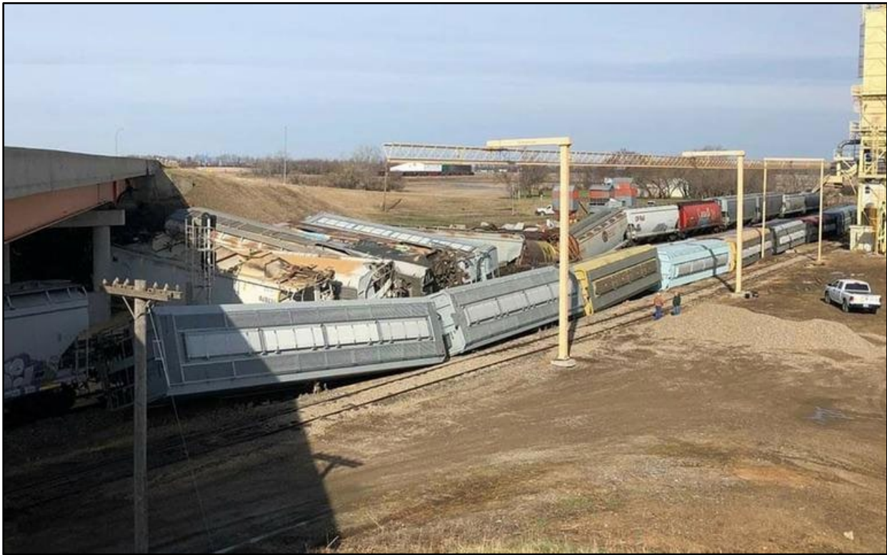
Figure 4.14.1 – April 26, 2020, Train Derailment at the City of Carrington
