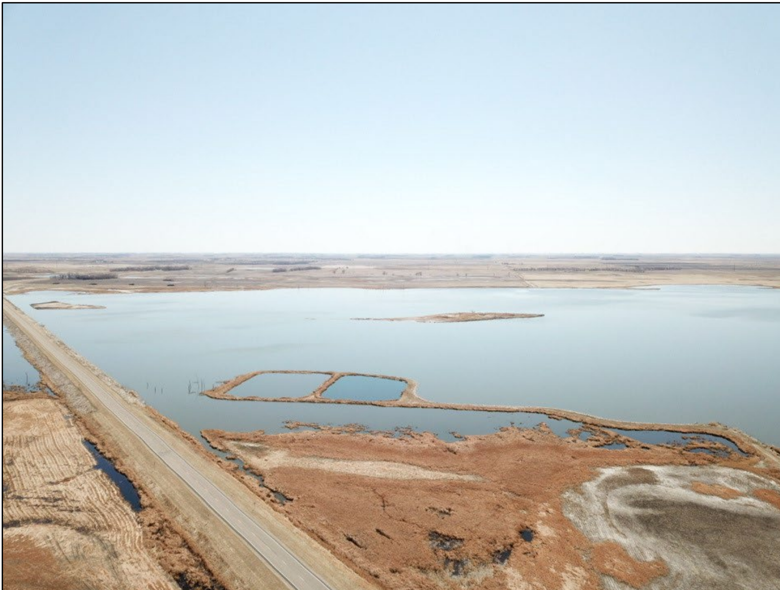
Figure 6.1 – City of McHenry Sanitary Sewer Lagoons
