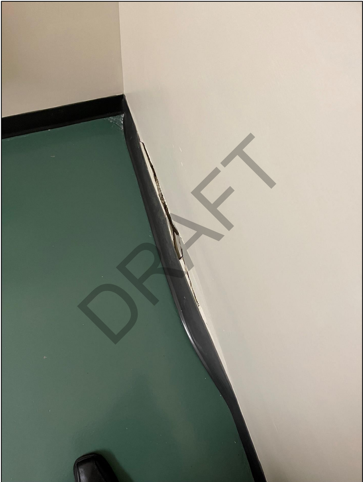
Figure 6.4 – Foster County Courthouse Substructure Heaving #1
