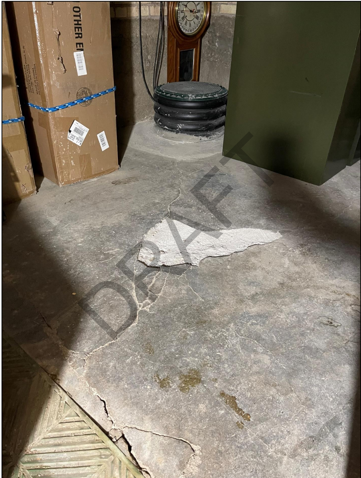
Figure 6.2 – Foster County Courthouse Substructure Heaving #1
